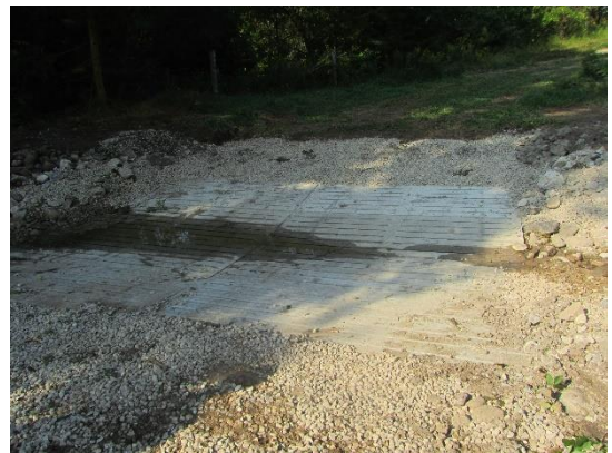
Example of Hog Slot Low Level Crossing
